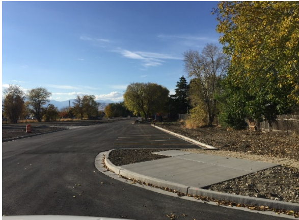
Infrastructure for future 26-unit senior project in American Fork.
